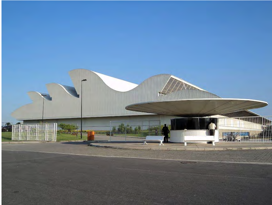
Fig. 80 Acceso principal con caseta de control. Panoramio – Google Maps. http://www.panoramio.com/?no_redirect - Photos by RNLatvian
