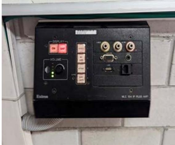
**Image 6.** Control panel for projector and retractable screen.
